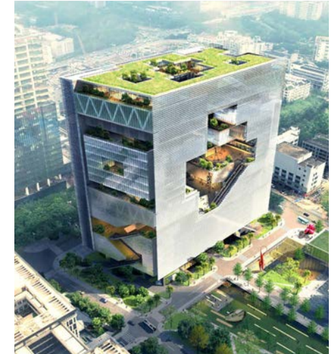
Shenzhen New Cultural Centre Futian, China
