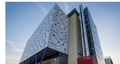
Data Centre - East London London, United Kingdom
